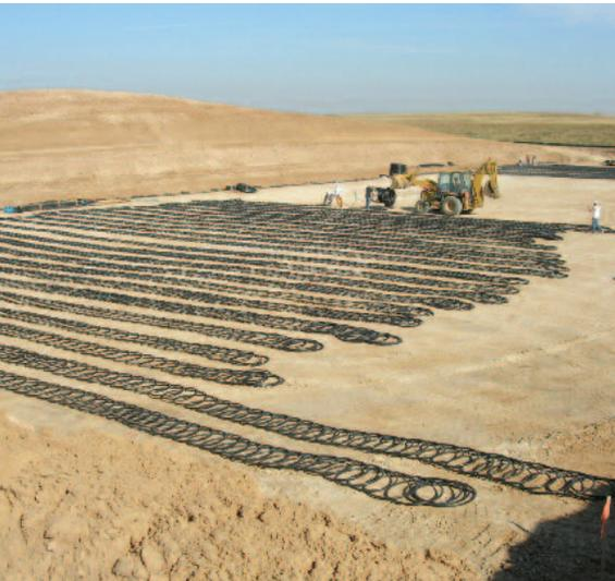
Installation of the geothermal system. Piping buried beneath the earth exchanges heat between the earth and building to provide year-round heating and cooling. *Photo - M.E. GROUP*
